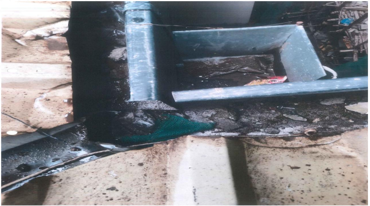
Figure 7: Pictorial representation of building debris deposited on the roof of Coldstone Building
